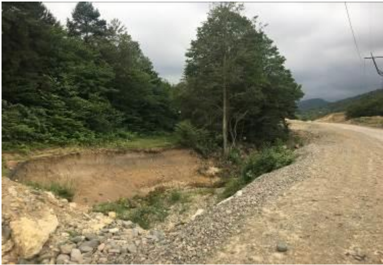
Deep cuts, trenches and pits, are without relevant barriers and warning signs
