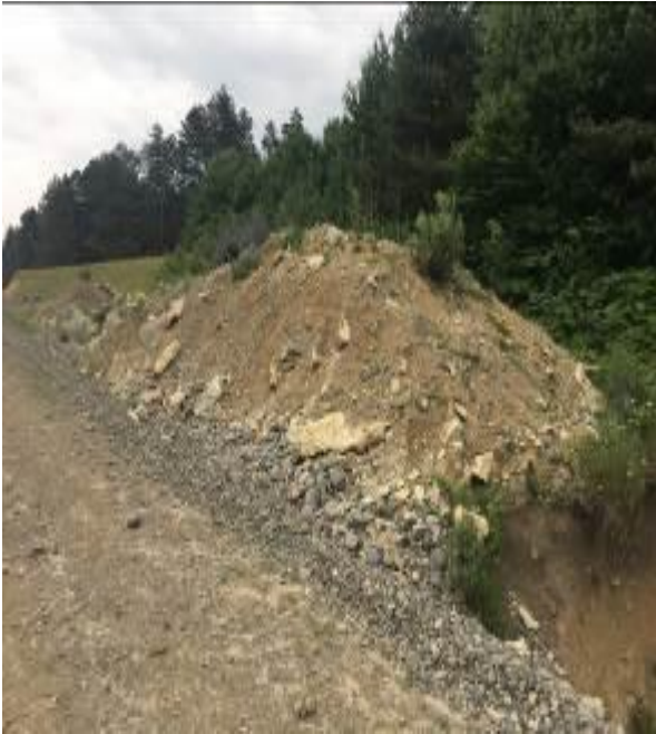
Deep cuts, trenches and pits, are without relevant barriers and warning signs
