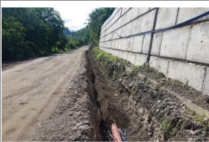
Km 12+870 ~ km 12+900: Backfill with Sand
