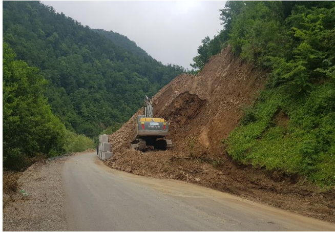
Km 20+000 ~ Km 20+250 (RHS):Excavation of Slope
