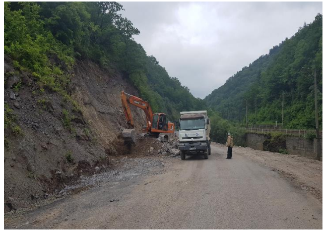
Km 24+080 ~ km 24+180 (LHS):Excavation of Slope
