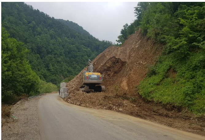
Km 20+000 ~ Km 20+250 (RHS):Excavation of Slope
