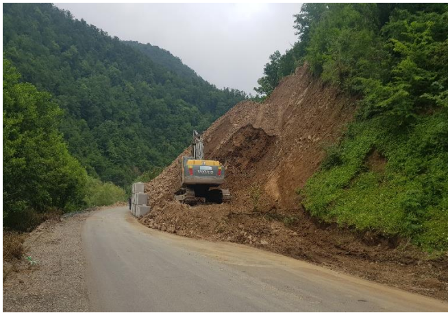
Km 20+000 ~ Km 20+250 (RHS):Excavation of Slope
