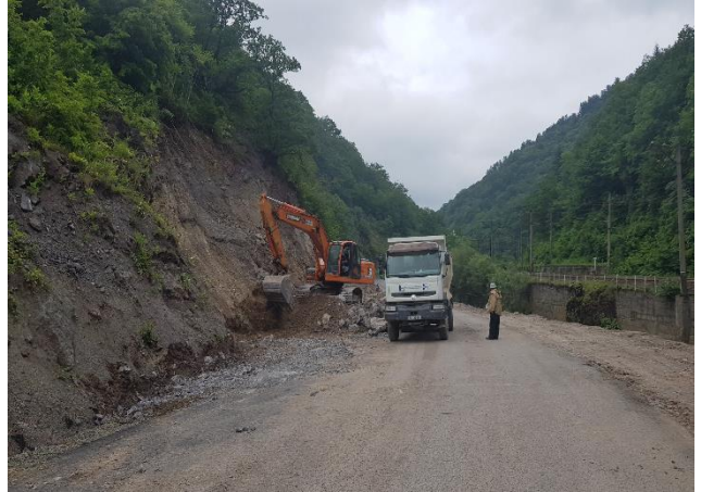
Km 24+080 ~ km 24+180 (LHS):Excavation of Slope
