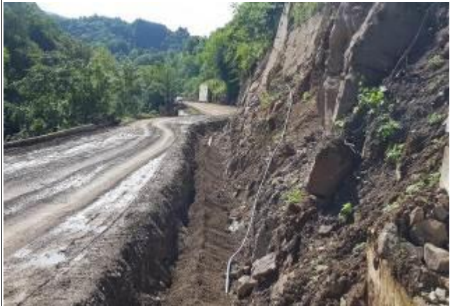
Km12+900 ~ Km13+310: Backfill with Sand
