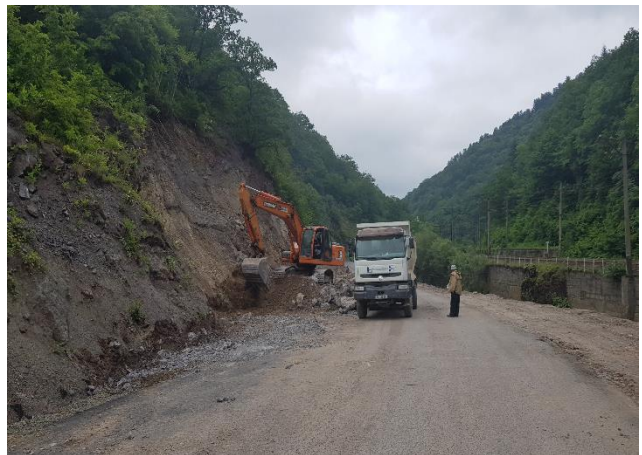
Km 24+080 ~ km 24+180 (LHS):Excavation of Slope
